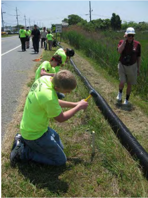
Student interns install barrier fences along the causeways to prevent turtles from entering the road.
